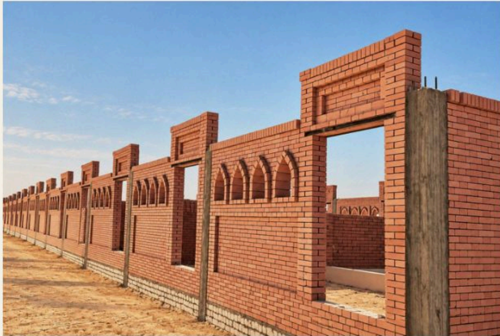
Fair-faced brick walls of the cemetery blocks
