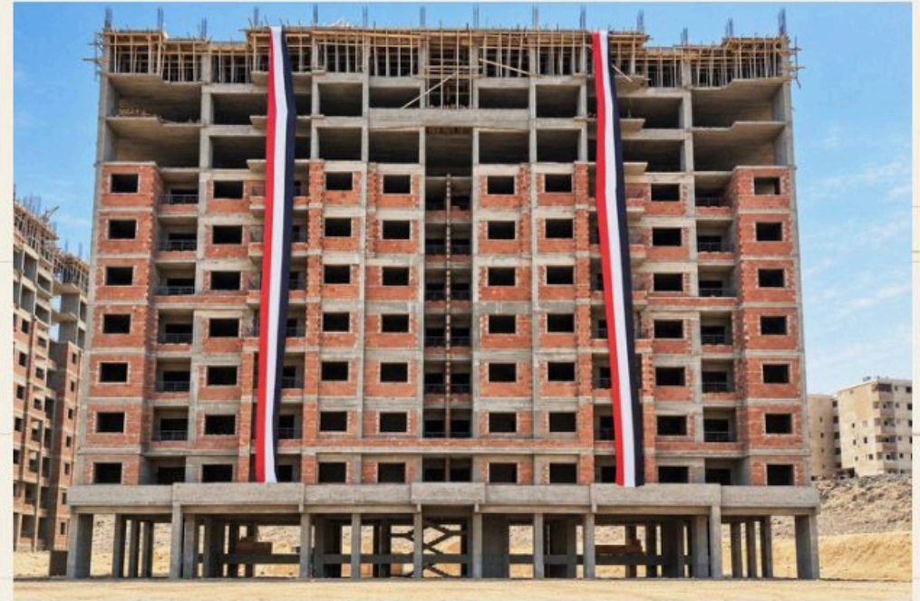
Concrete-frame stage — on site
