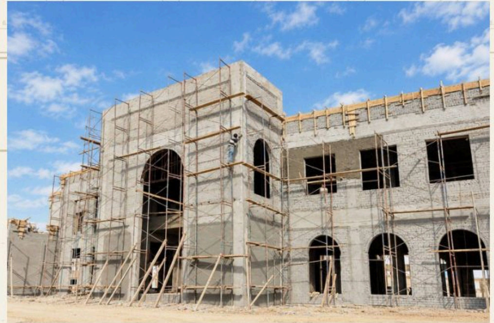
Main façade during plastering — on site
