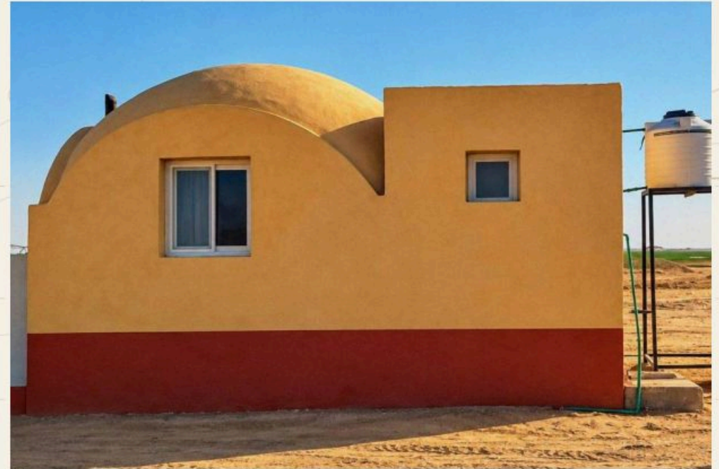
One of the 163 centre-pivot control rooms
