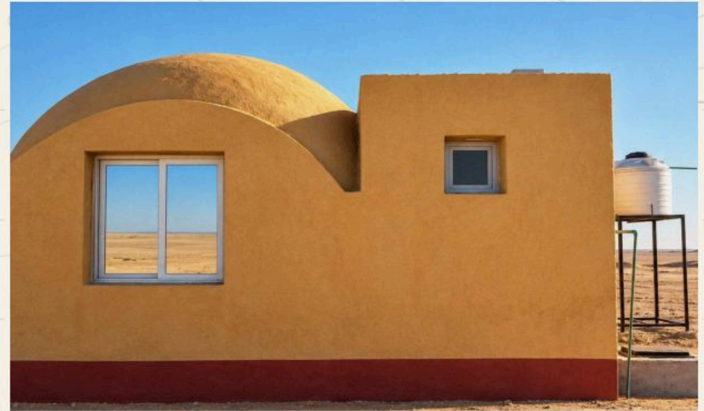
Control room — on site
