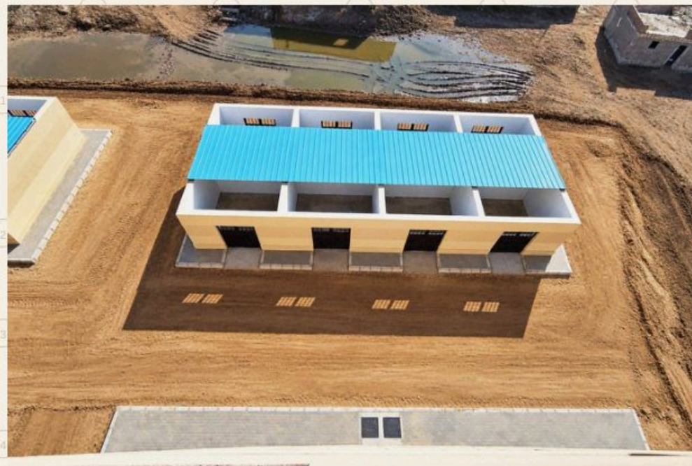
Livestock barns — on site
