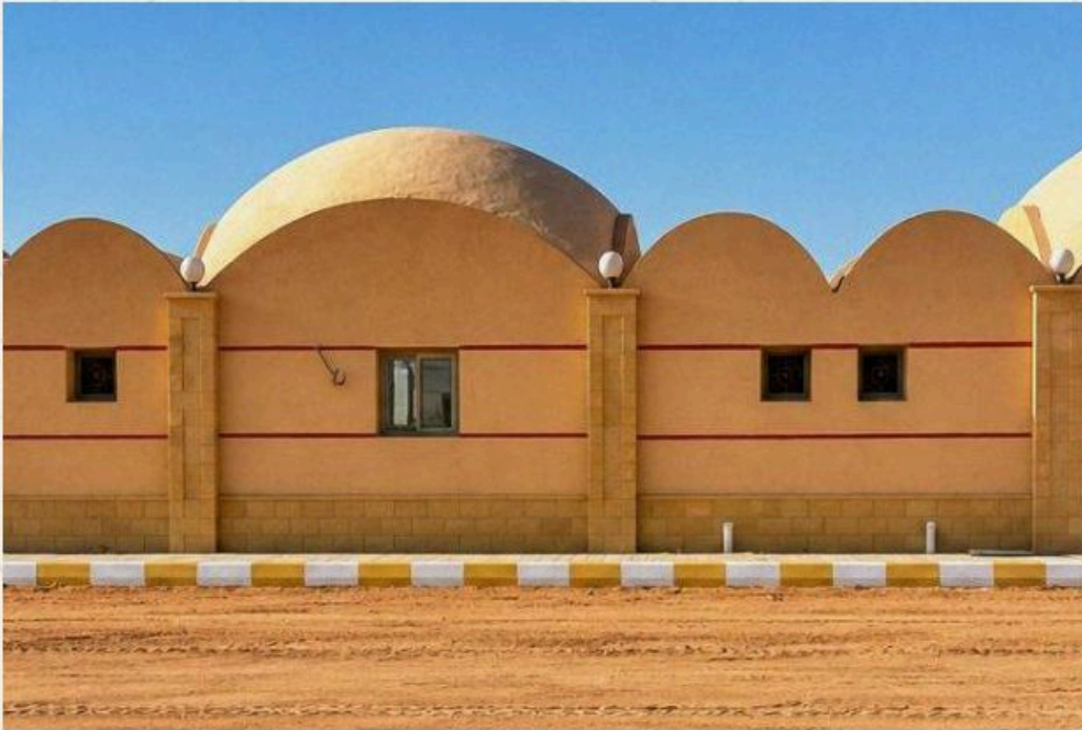
The administrative and residential compound
