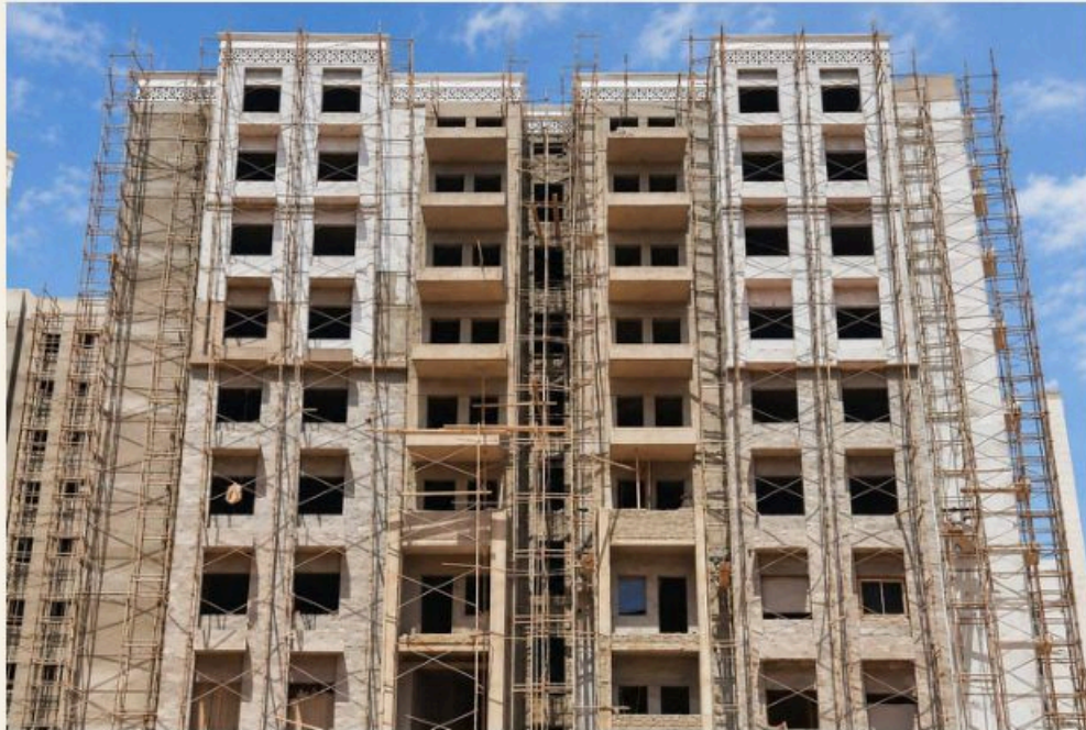
Façades in progress
